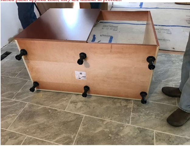
**3.** Start in corner and work out of corner putting cabinets in place and adjust back of cabinet up to level line on wall (you can use a <u>long flat head screwdriver</u> to adjust back legs using the slots in the foot of the leg), then plumb cabinet with front legs, clamp together with quick clamps and screw cabinets together using 1-1/4" screws.
